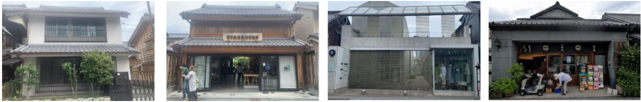
Figure 4-2: Newly Constructed Buildings
