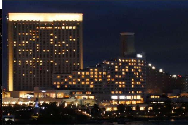
Figure 5: Building View (C32) Hilton Hotel Odaiba, weekend, 19:54.
